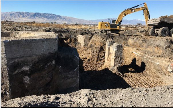
Excavation and removal of contamination
