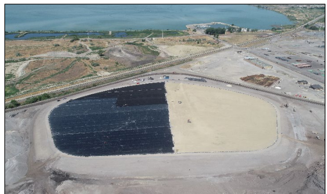
Aerial view of corrective action management unit (CAMU)
