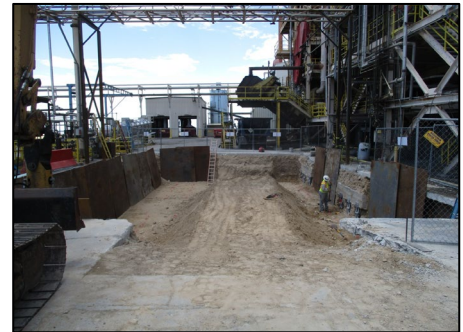
Early stages of construction of the shredder foundation
